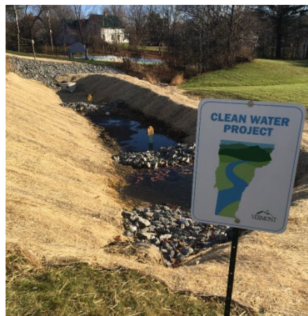
Figure 30. Before (left) and after (right) the conversion of a paved swale into a gravel wetland to treat runoff from the parking lot at the Hazen Union School in Town of Hardwick. Project funded by a DEC Clean Water Initiative Program grant. (Source: Caledonia County Natural Resources Conservation District)
