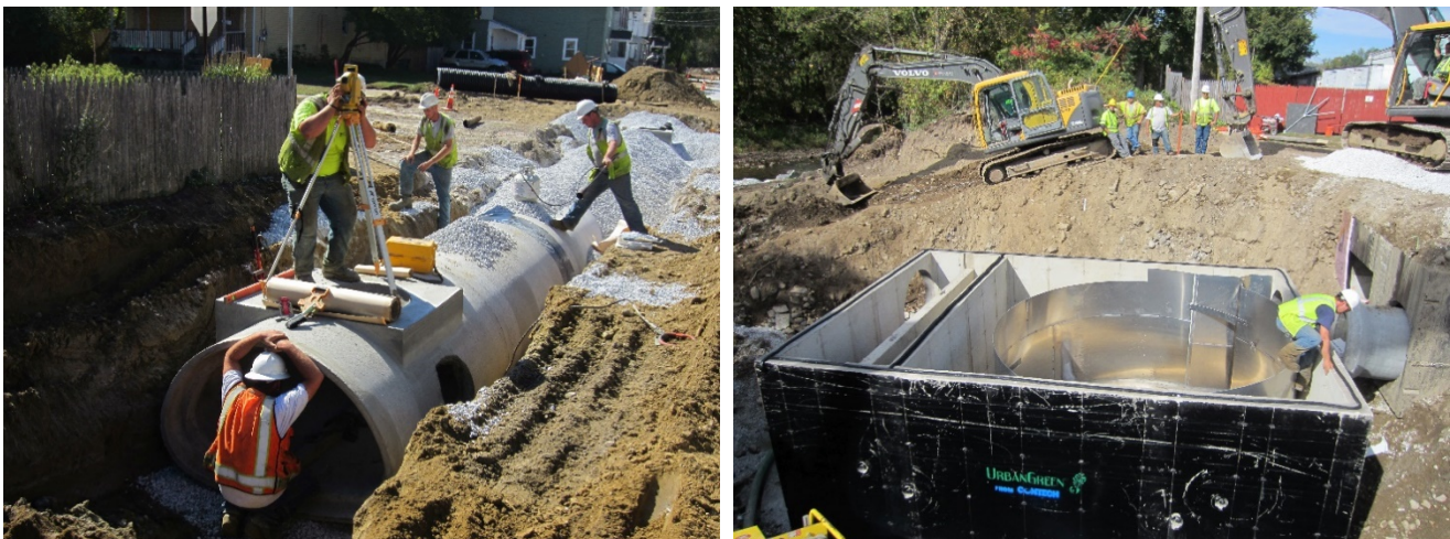
Figure 32. Installation of a reinforced concrete pipe (left) and stormwater separation system (right) to abate combined sewer overflows (CSOs) in the City of Rutland. Project financed by the Clean Water State Revolving Fund. (Source: Otter Creek Engineering)
