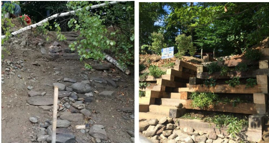
Figure 36. Before (left) and after (right) the installation of Vermont's first crib-wall staircase to remediate erosion at a lakeshore access point in Waterbury Center State Park. Project funded by DEC Clean Water Initiative Program grant. (Source: Vermont Youth Conservation Corps)
