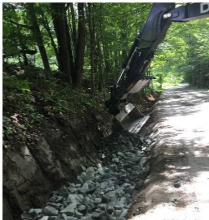
Figure 31. During (left) and after (right) the construction of stone-lined drainage ditch in the Town of West Windsor. Project funding provided by VTrans Better Roads Program. (Source: VTrans)
