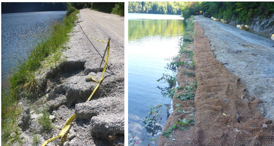
Figure 34. Before (left) and after (right) the installation of encapsulated soil lifts to naturally stabilize and reduce erosion along Black Pond Road in Town of Hubbardton. Project funded by a DEC Clean Water Initiative Program grant. (Source: Northwoods Stewardship Center)
