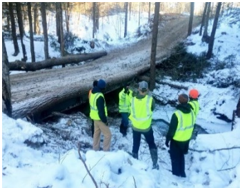
Forester training on temporary skidder bridges at Mount Mansfield State Forest
